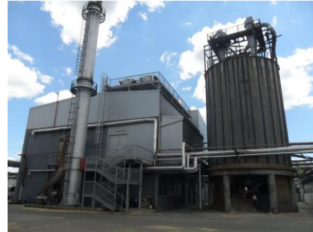
Figure 1. Biomass CHP biomass power plant Spin Valis International
